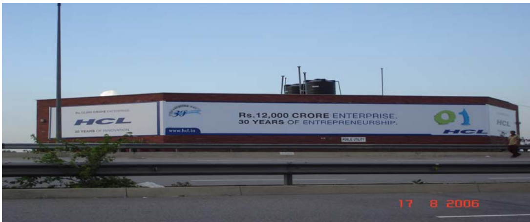
Panel on Toll Plaza Building
