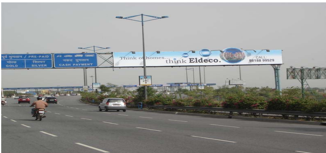
Panel on Back Side Of Gantry
