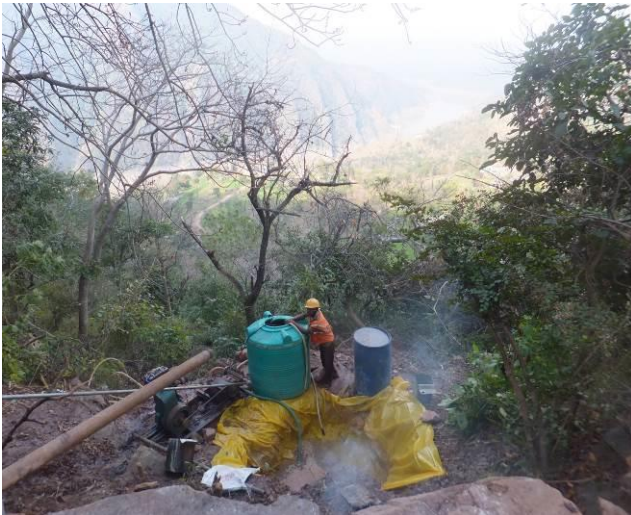
Figure 2. Tunnel 1, portal 1 – Borehole 4 Location.
