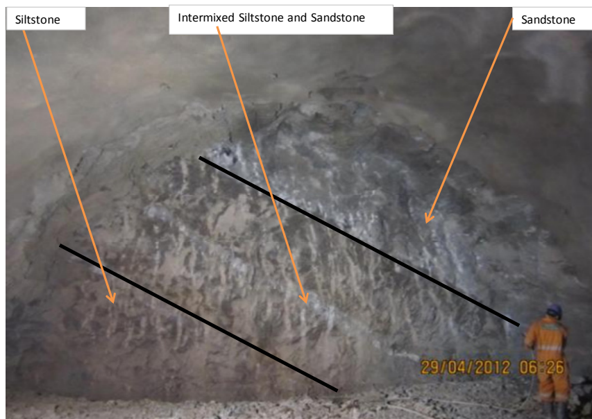
Figure 2. Photo showing exposure of different rocks at one location in main tunnel, south end
