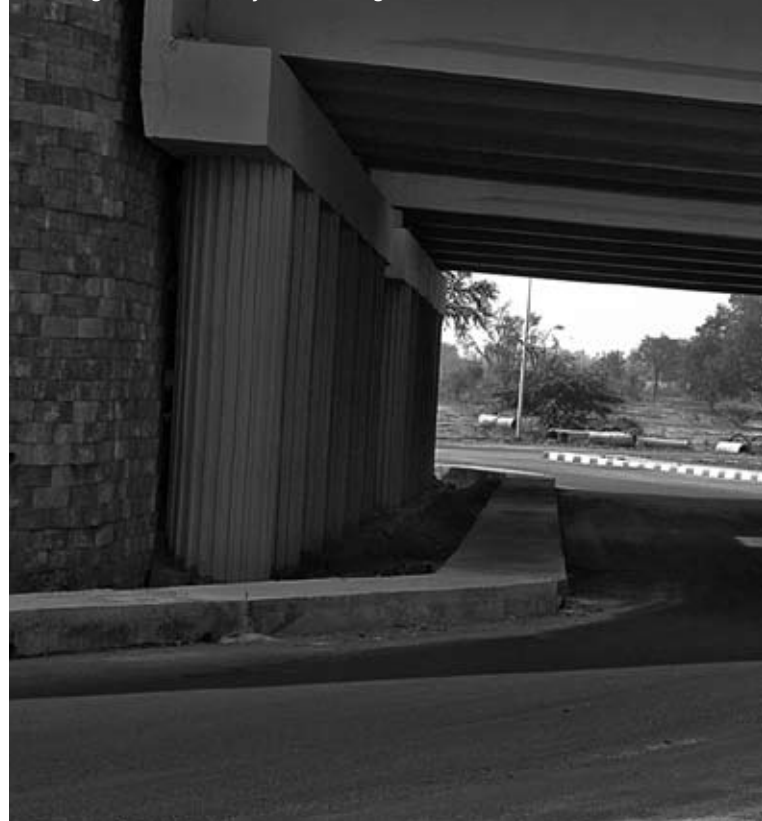
Vehicular Underpass at Peddagolkonda Rotary Interchange
