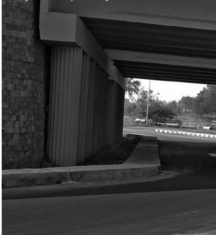
Vehicular Underpass at Peddagolkonda Rotary Interchange
