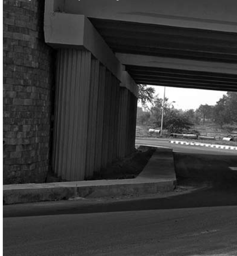
Vehicular Underpass at Peddagolkonda Rotary Interchange
