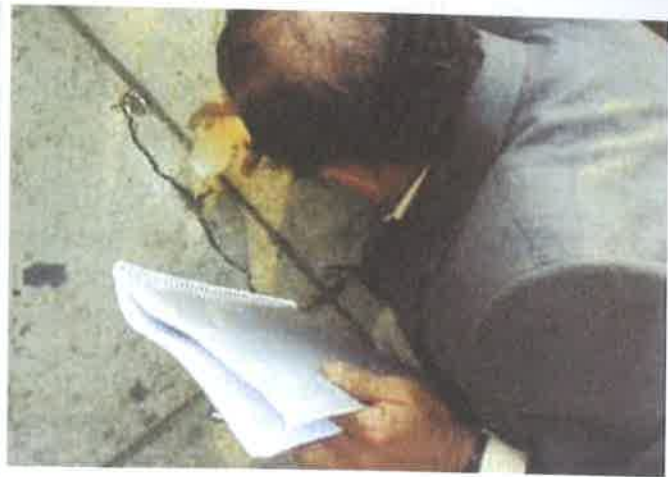
Pouring Low Viscosity Epoxy Resin
