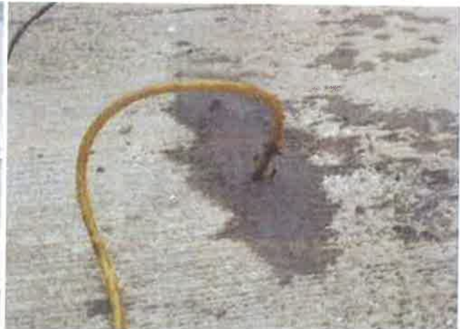
Treatment of Shallow Spalling at Joints by Gravity Sealing with Low Viscosity Epoxy
