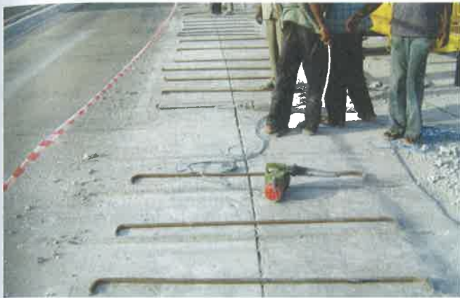
(a) Slot Cutting and U-Shaped Staples
