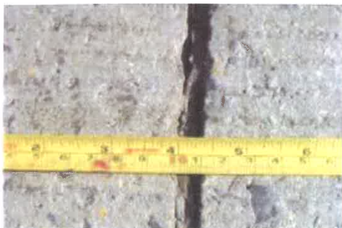
b) Sand blasting the groove after raking out the sealant residue and rubbish from the joint.
