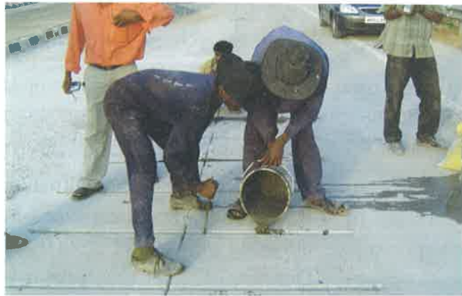
(b) Slot Filled with Elastomeric Concrete
