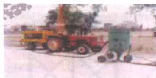
b) Sand blasting the groove after raking out the sealant residue and rubbish from the joint.
