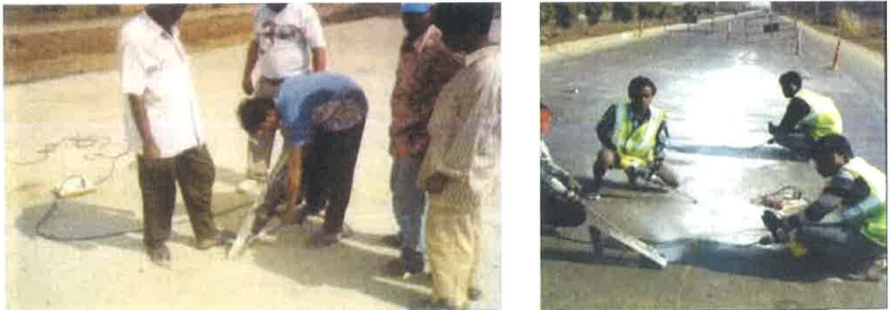
Fig. 7.2 Drilling Inclined Holes with Angle Template
